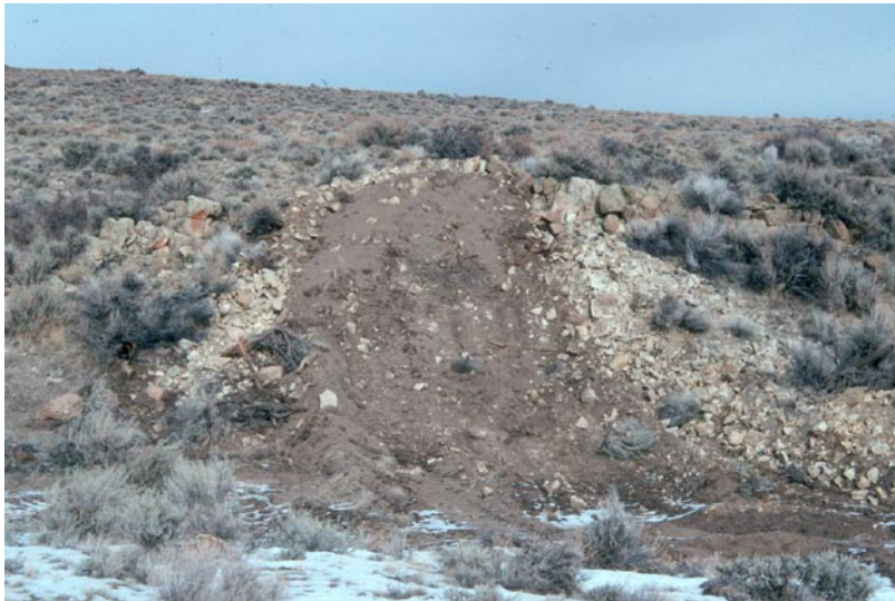
Sealing of a mine and former winter roost site, Ellen D. Mountain, Elko Co. Photo by Pete Bradley.
